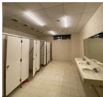
緣起樓 B1 廁所改 LED 支架燈
